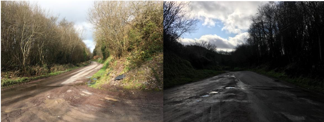
Plate 4-4: Views from Site Entrance Looking North and South
