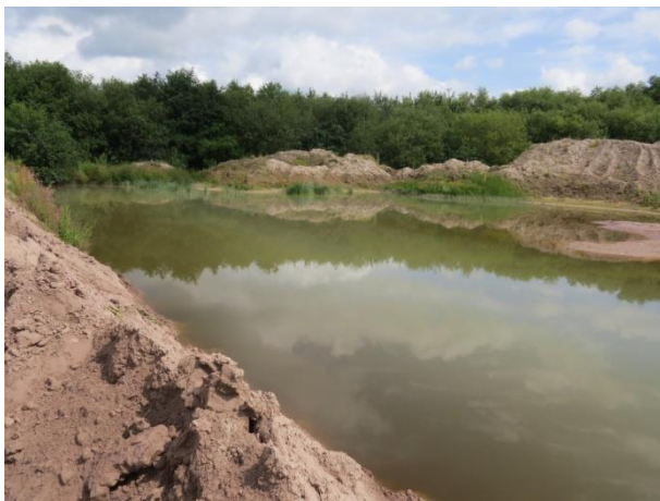
Plate 10-16: Western Settlement Pond (July 2019)
