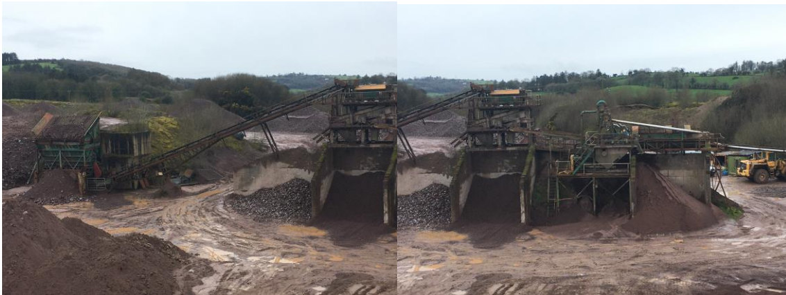
Plate 2-1: View of Washing Plant from the East
